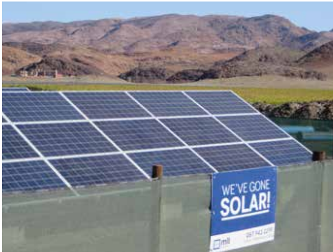
New solar panel project at SVL
