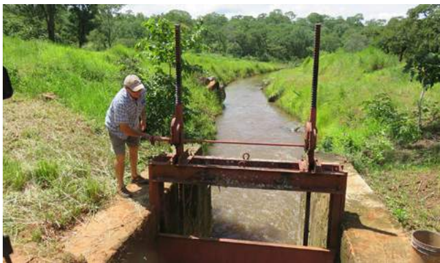
A weir controls water offtake from the river into a canal (left). Water then flows into a pipe, which drops steeply down a bank and into the turbine house (right).
