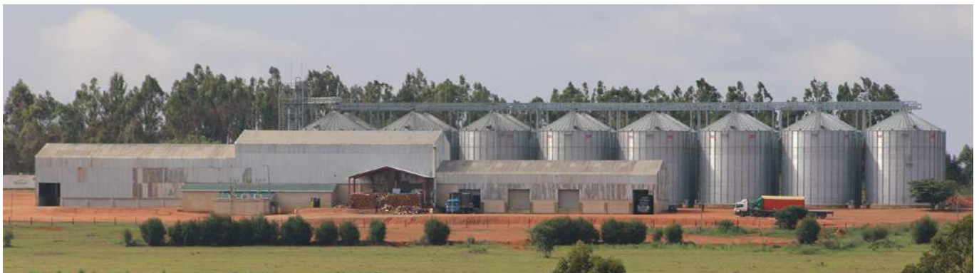
The Silverlands Tanzania feed mill housed in the shed with silos behind.
