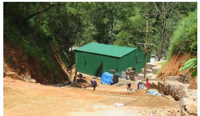
A weir controls water offtake from the river into a canal (left). Water then flows into a pipe, which drops steeply down a bank and into the turbine house (right).
