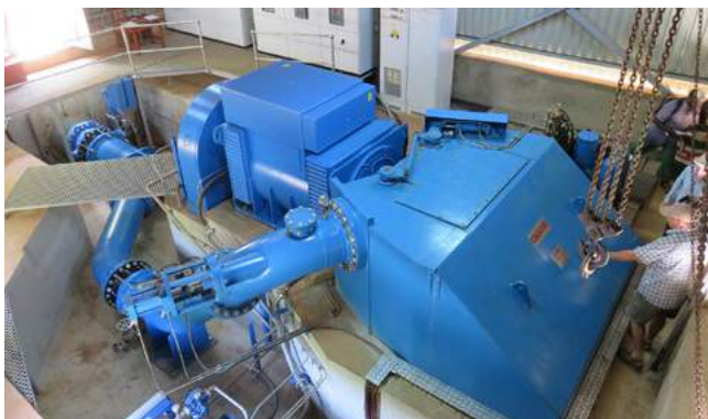
Water enters from the left and turns turbines in the large blue casings (left), before being released back into the Ruhuhu River (right).
