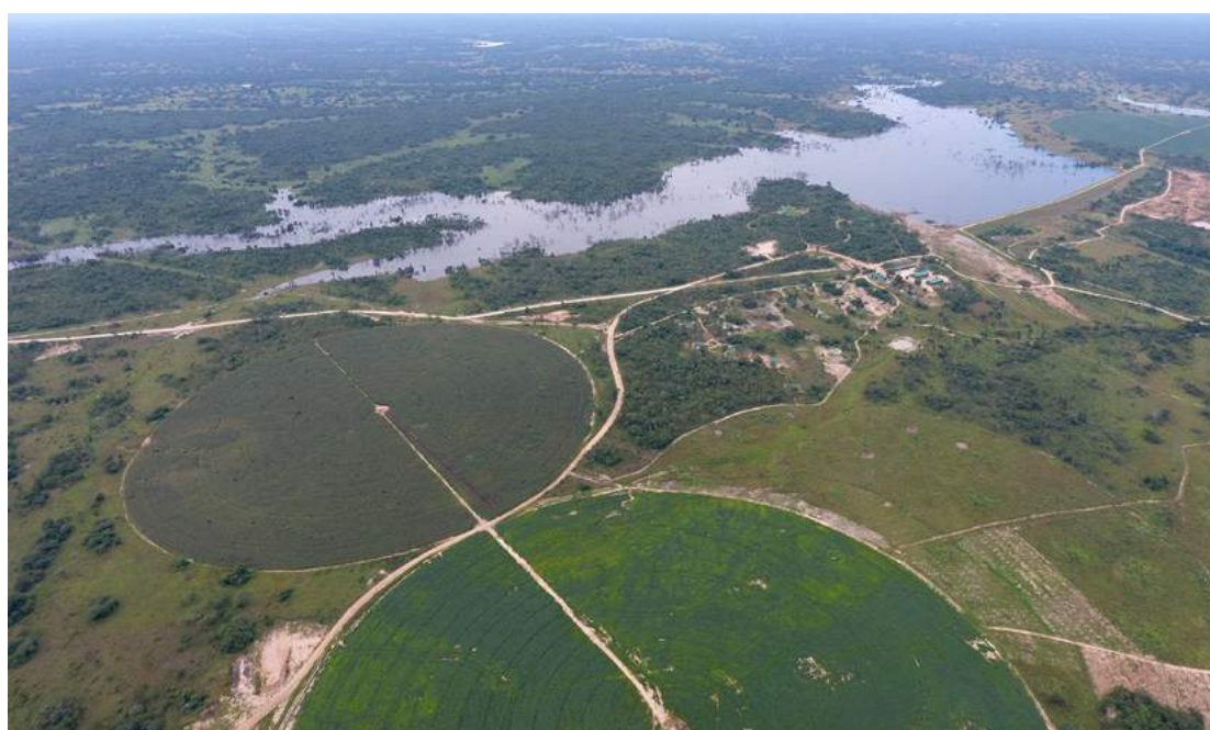
The new 'hub' of Silverlands Ranching, including 13m 3 dam, cropping, housing, offices, stores and workshop.
